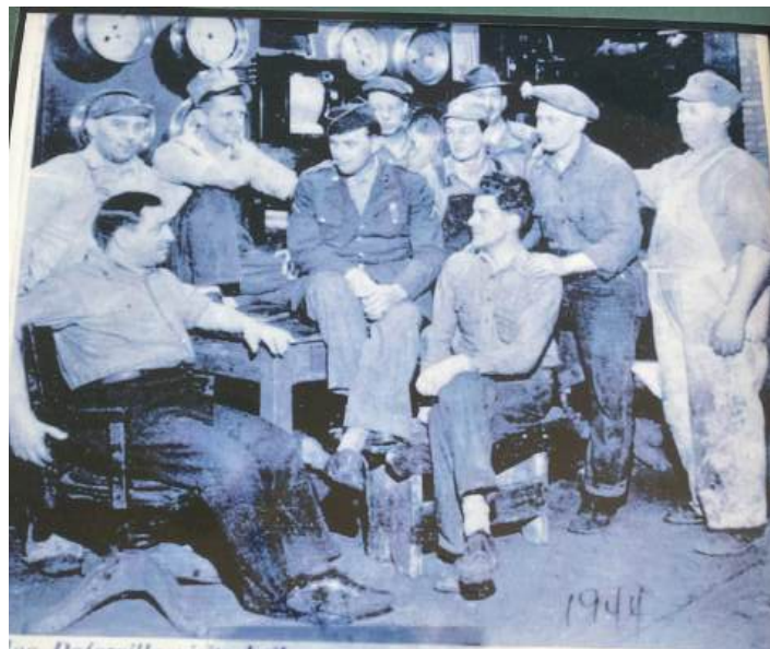
Joe Deferville visits boiler room gang (6)
