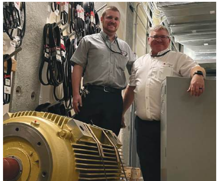
Frank Gallina and Cory Lane with redundant building equipment — a spare motor and disconnect.
