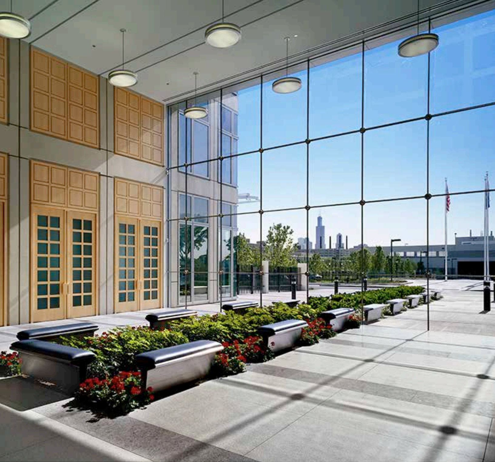
The building's lobby features a glass wall maintained via a cable net structure that offers expansive views of the Chicago skyline. (Photo: ©David Seide/DefinedSpace.com)
