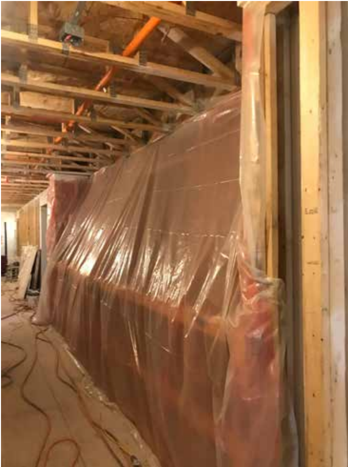
A containment area in a newly built environment.
