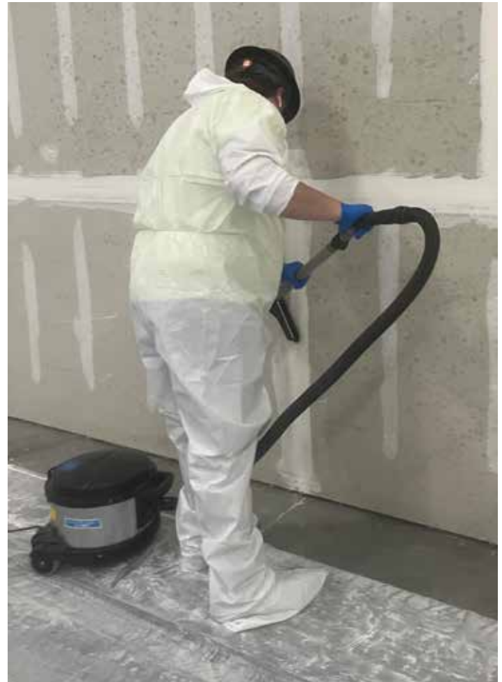
Sanding drywall at a facility with a dustless HEPA vacuum system.
