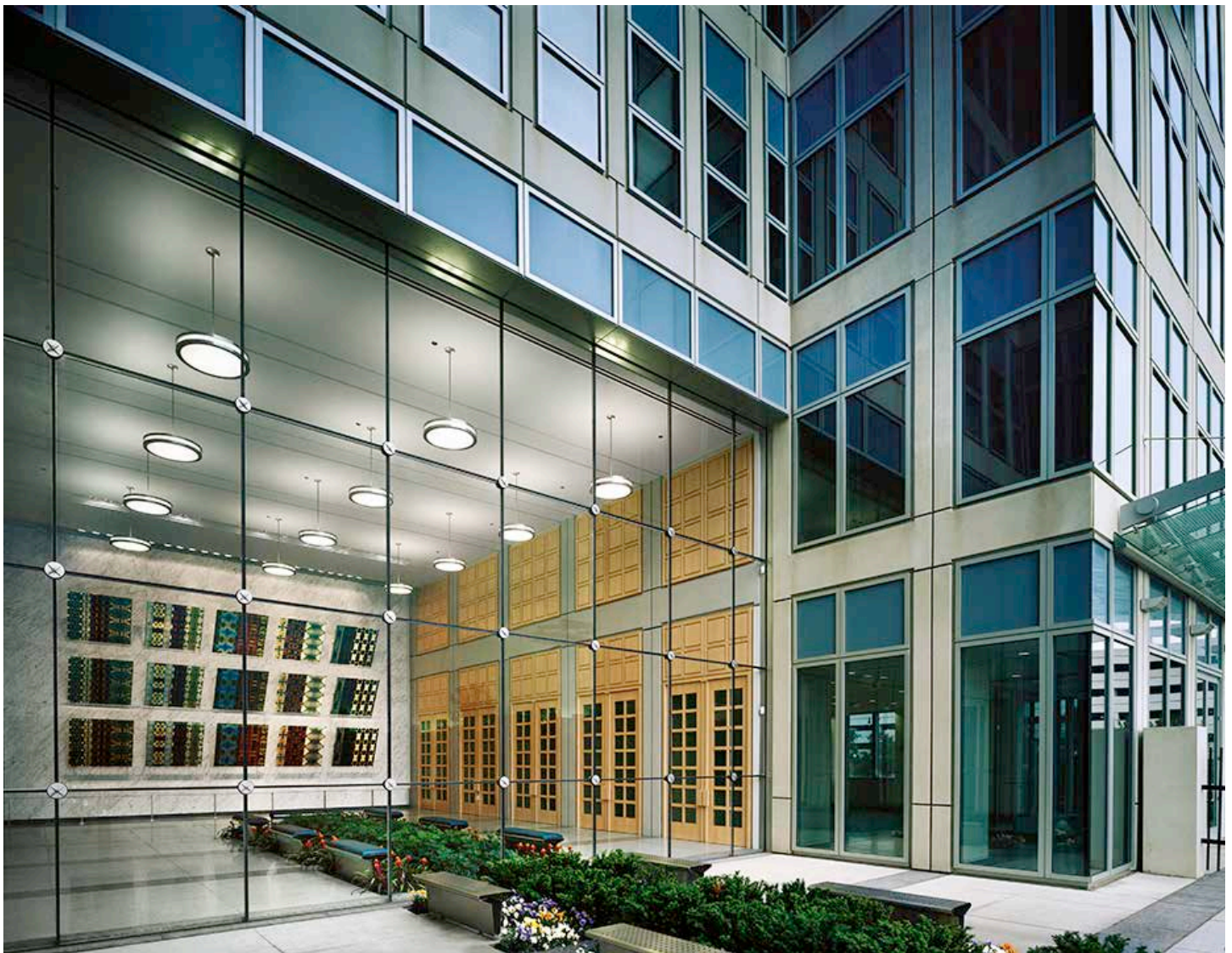
The façade and exterior wall of the FBI Chicago Regional Office is composed of about 60 percent architectural precast concrete, and high-performance, low-E glass, making for a very energy-efficient envelope. (Photo: ©David Seide/DefinedSpace.com)
