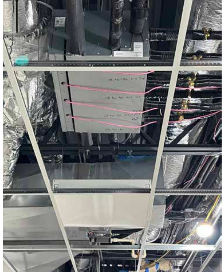
A four-port refrigerant branch unit in the foreground with a high-static air handler in the background.
