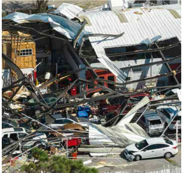
As severe weather and wildfires become more frequent, Schneider Electric is developing new tools to help utilities strengthen grid resilience, limit power outages, and restore service faster when the system comes under strain.
