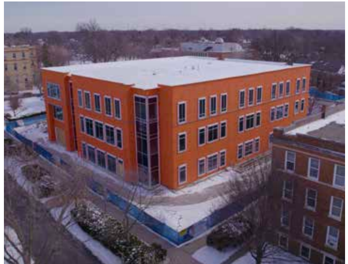
Cyclone Energy Group was instrumental in Elmhurst University's Health and Sciences Building earning its recent LEED Gold designation. (Photo: Elmhurst University)
