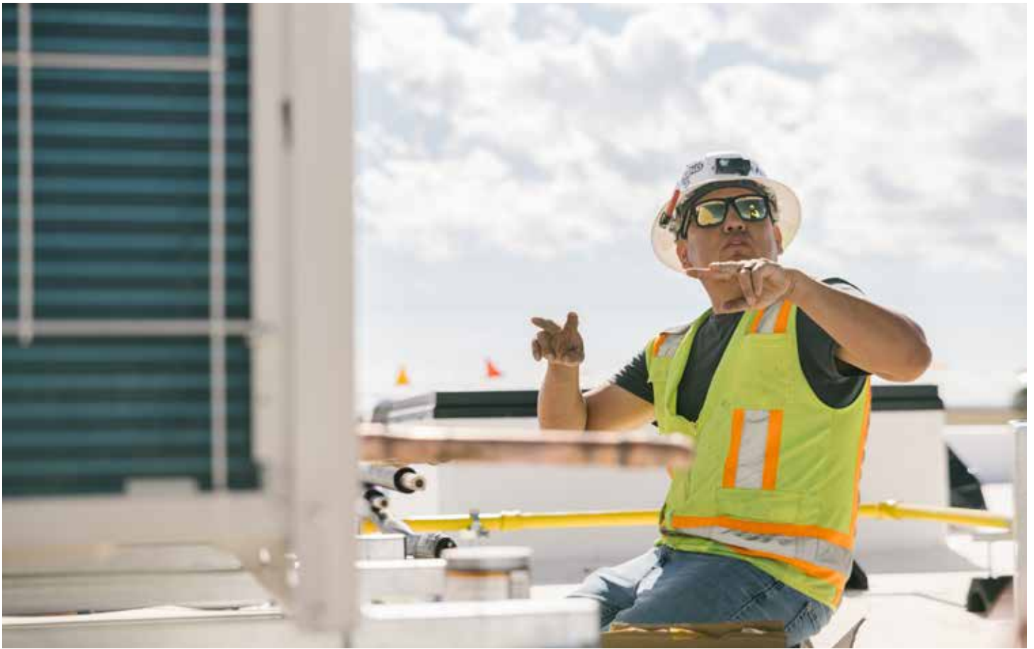
Foreman Jonathan John discusses heat recovery piping with a colleague.
