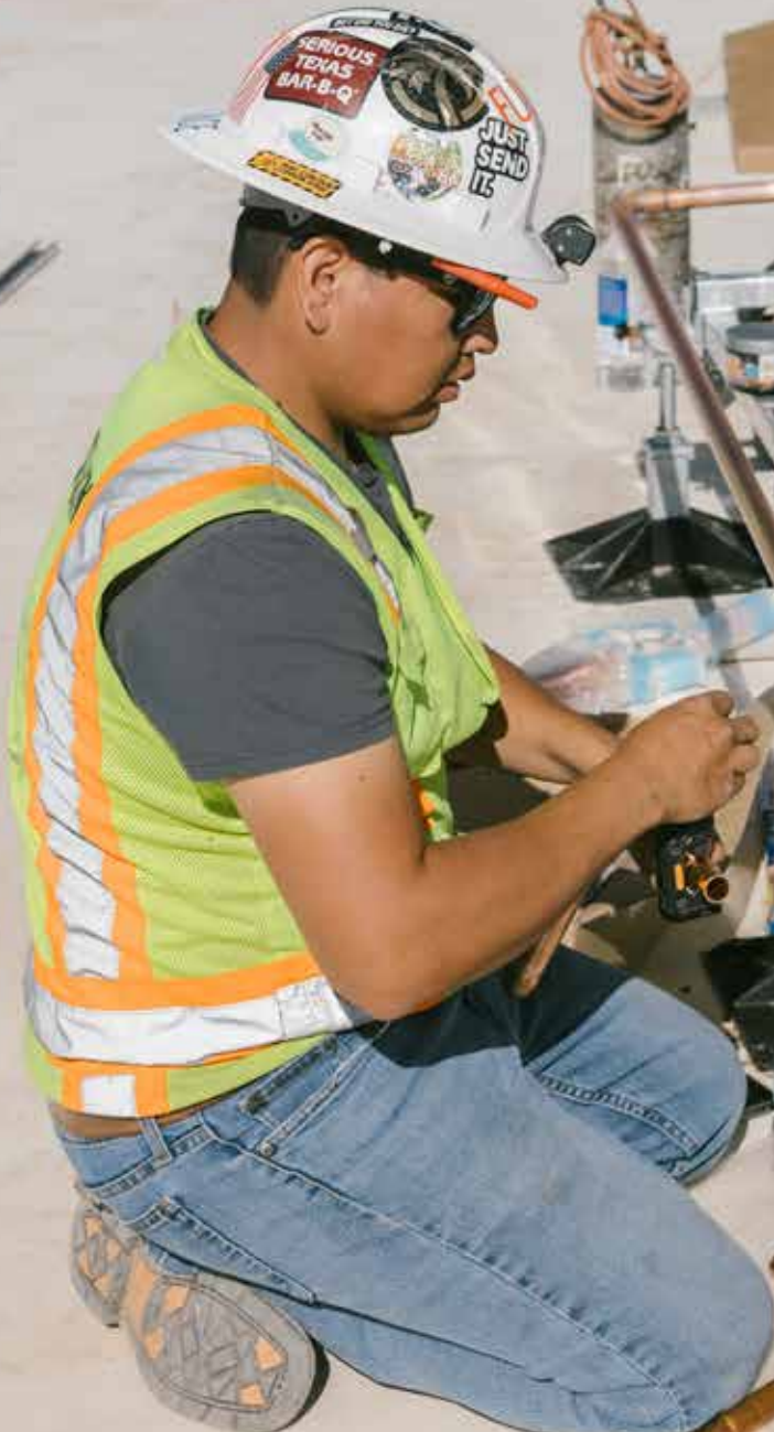
Foreman Jonathan John pipes a Fujitsu AIRSTAGE VU-V heat recovery system.
