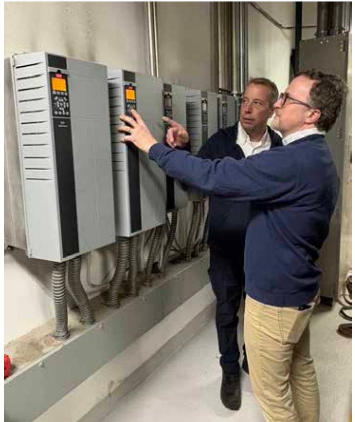
Keith Willburn and Nate Hultgren check out a set of Danfoss VFDs.
