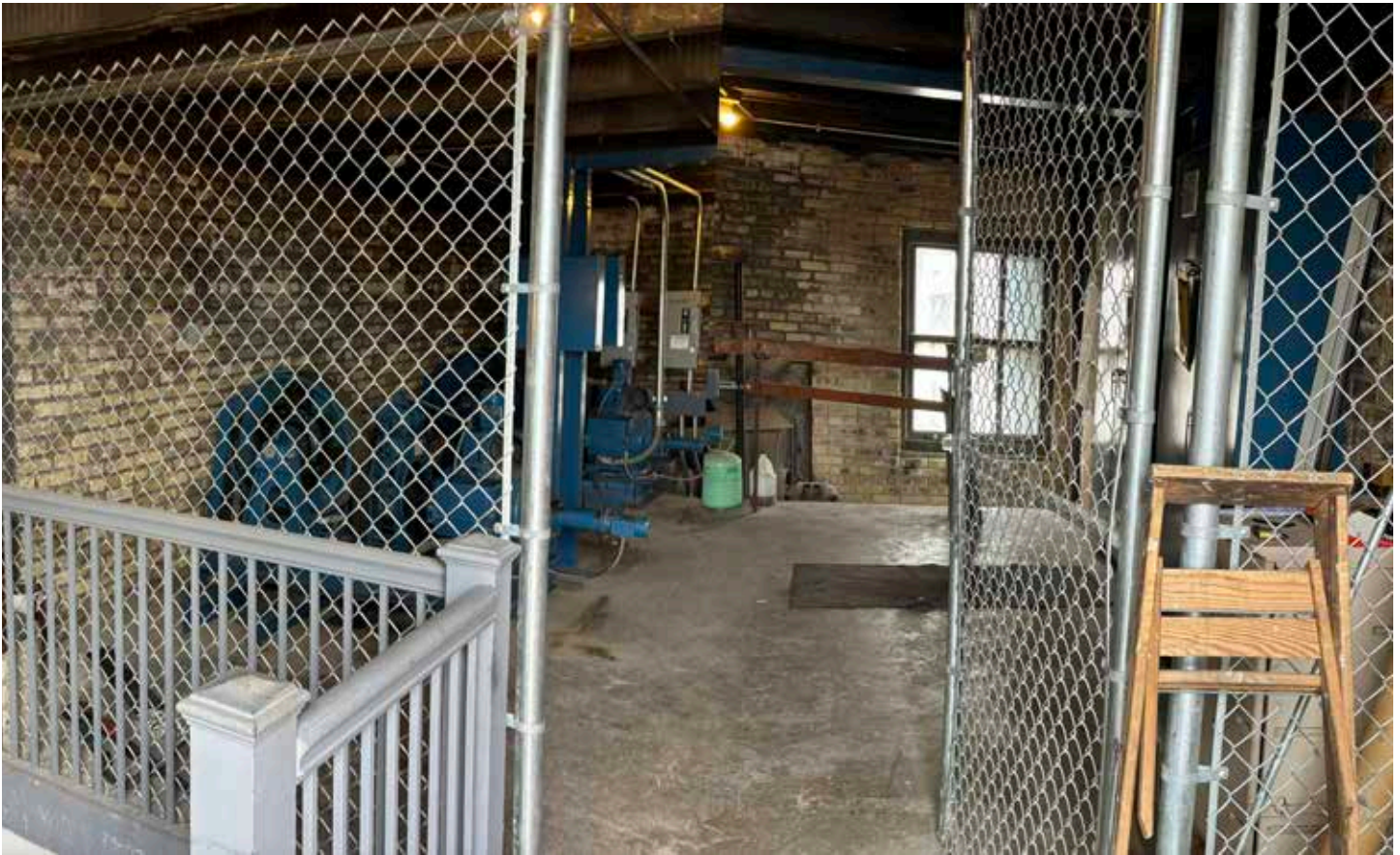
Elevator machine room prior to modernization.
