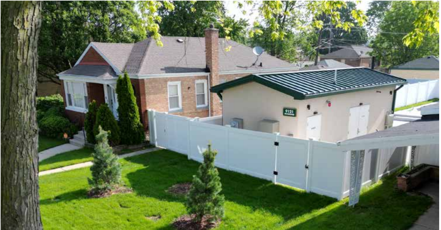
The lift station installed in Evergreen Park, Ill., was designed to blend in with its suburban surroundings.
