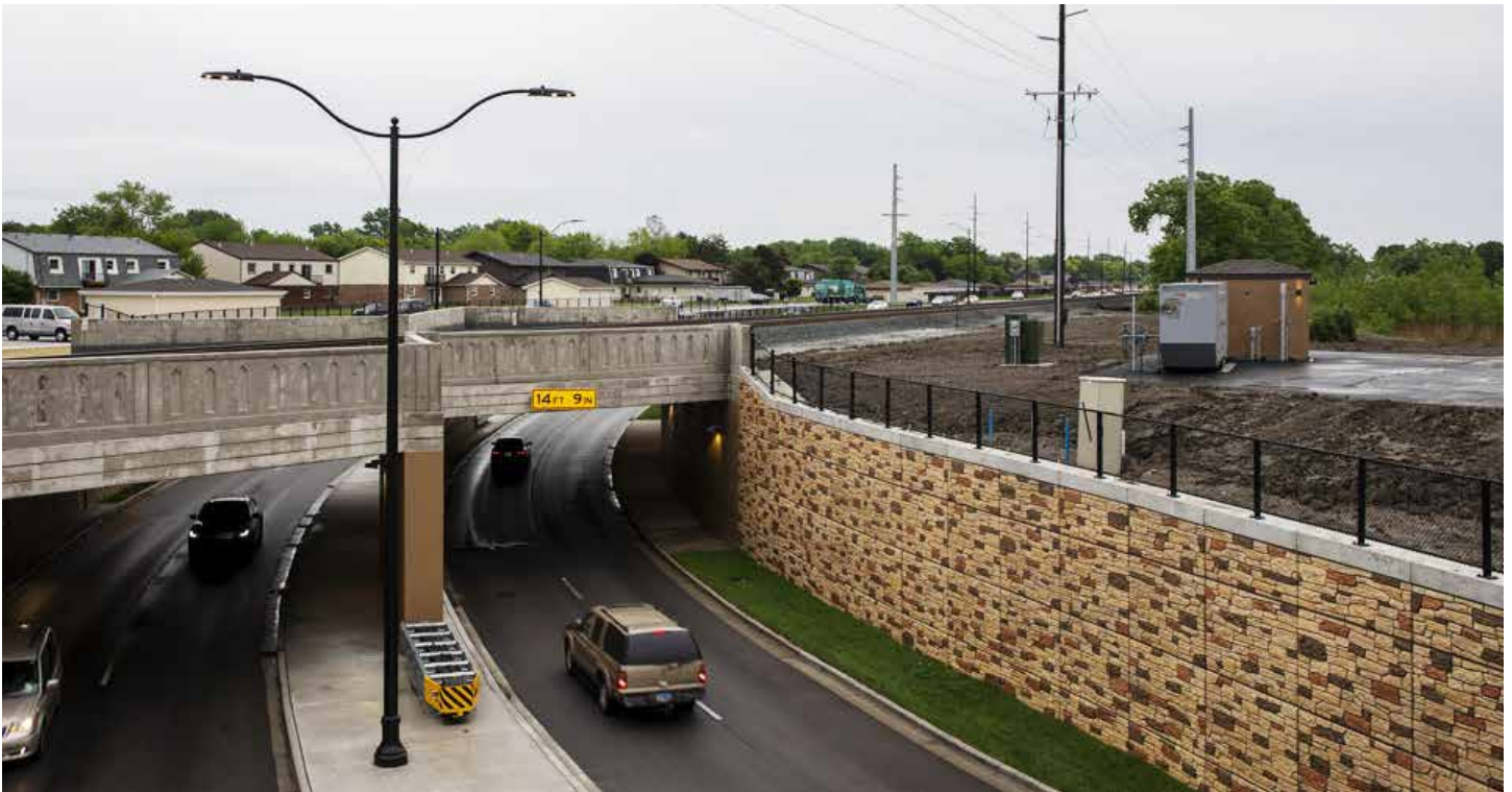
At right, the lift station in Munster, Ind., that manages storm water that otherwise might pool underneath the viaduct.
