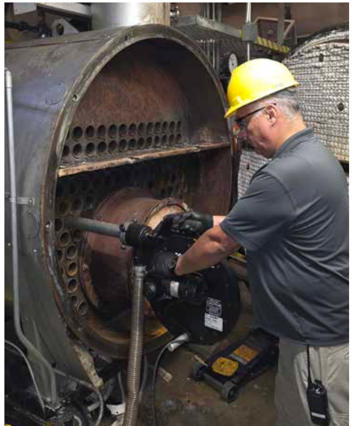
Alex Mendoza performs the annual boiler tube cleaning of the planetarium's Cleaver-Brooks firetube 250 hp. 2.
