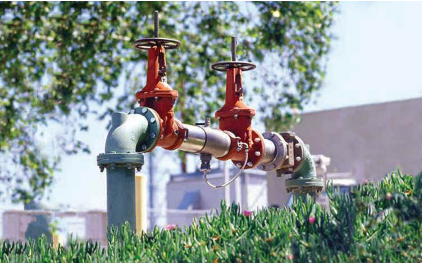
Commercial backflow devices protect public water supplies from contamination by preventing water from flowing backward from building into the municipal water main. Backflow assemblies act as a one-way valve, ensuring that water flows only in the correct direction, safeguarding public health by stopping harmful substances like chemicals, soaps, or industrial waste from mixing with clean, potable water.
