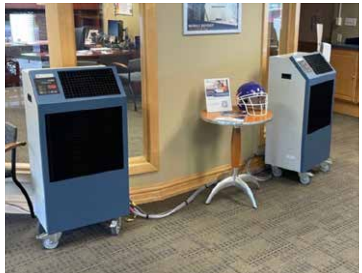
At 875 N. Michigan Ave., 1.5-ton, 115v water-cooled spot coolers are on hand in case of a tenant emergency.
