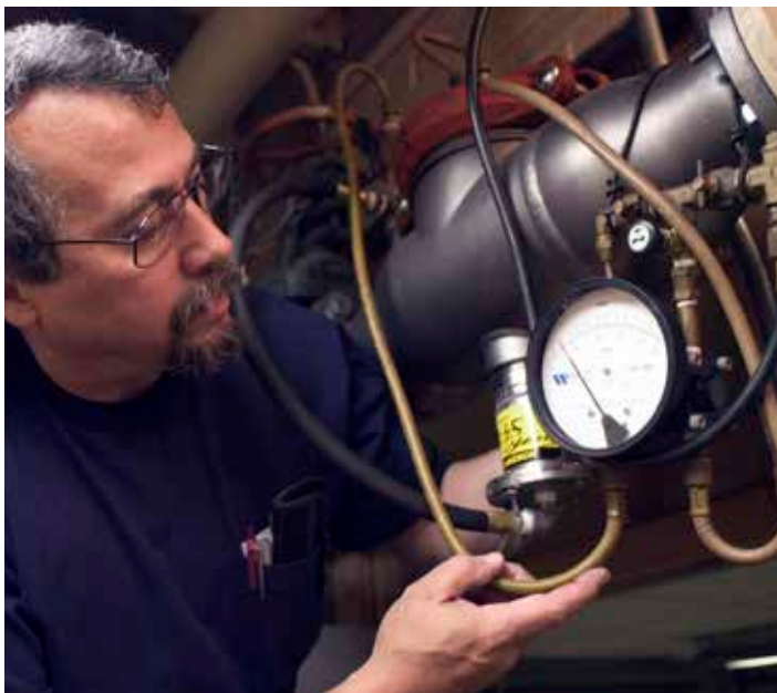
Annual testing is an important part of maintaining the performance of backflow assemblies.
