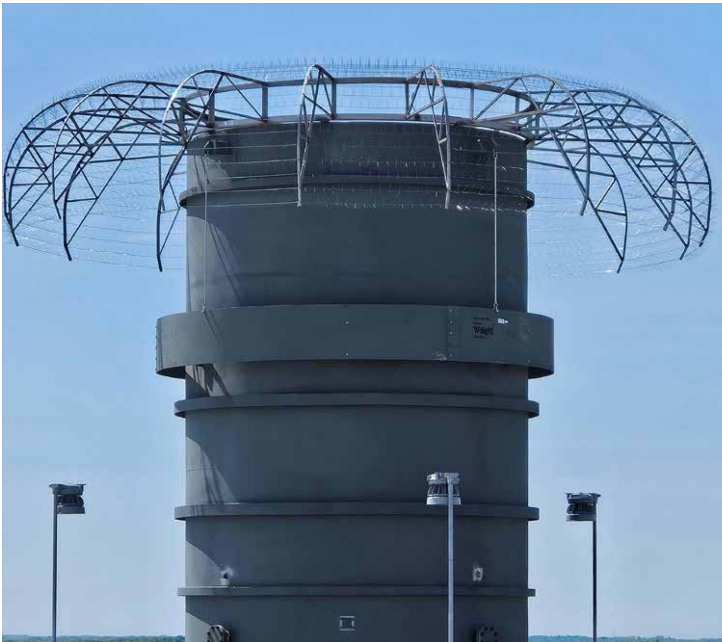
Considering the increasing risks posed by lightning-related events, power generation facilities cannot afford to rely on outdated or piecemeal lightning protection strategies.
