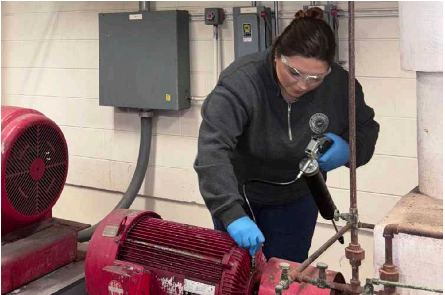
Kallie Fogarty greases one of many centrifugal chilled water pumps.
