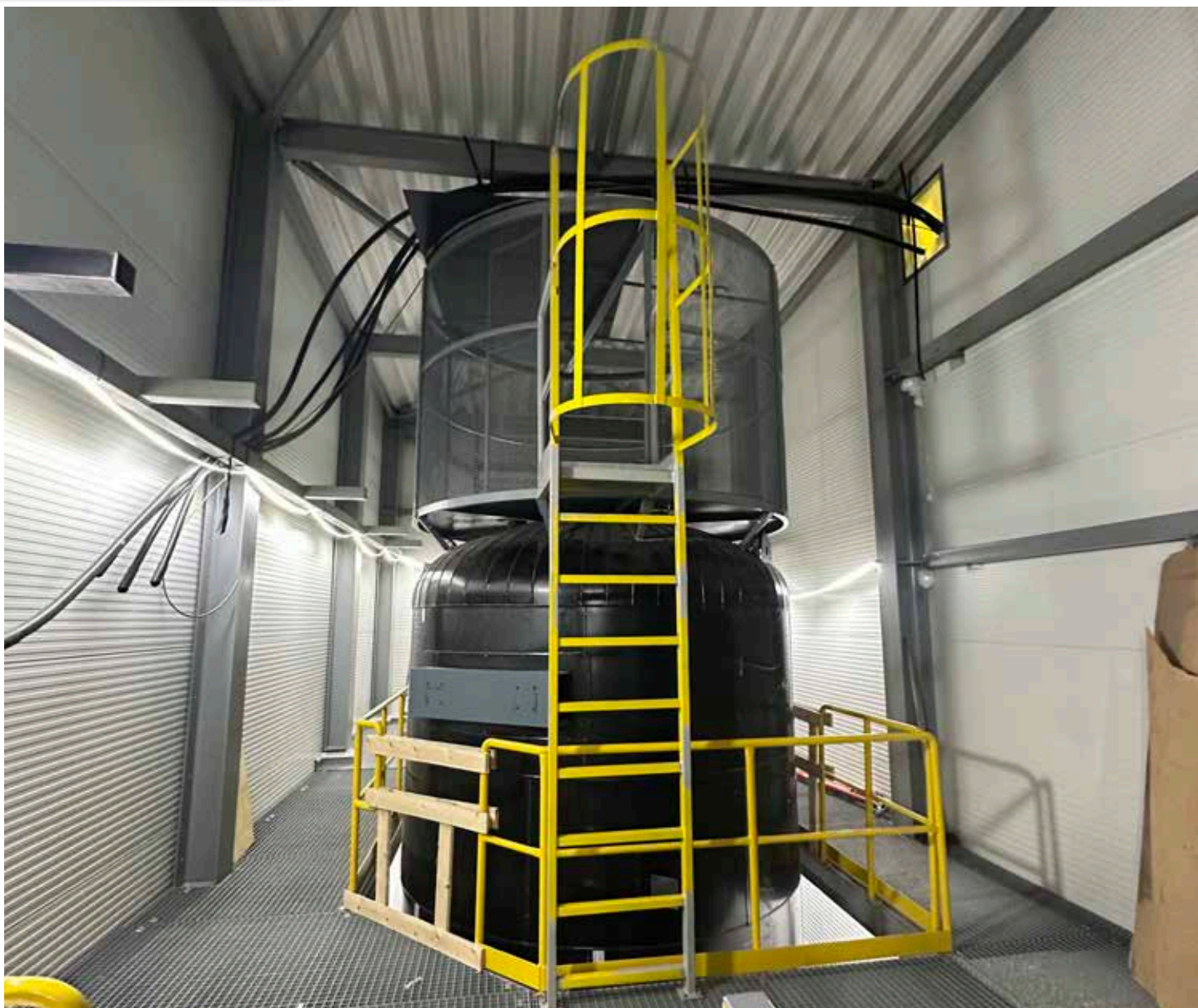
Modern high-output electrode boilers like those from Acme Engineering deliver zero emissions at the point of use, offer full modulation from zero to 100-percent output, and feature flexible configurations.
