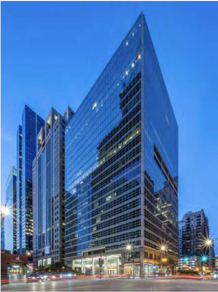
Mentorship from 101 North Wacker Chief Engineer Tim Maloney has allowed Tony to take on various building projects, including a demand-control ventilation strategy for operating the building's main air handlers.
