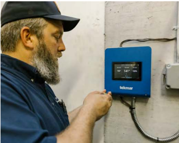
Kenny Walker, with Summers & Zims, installs the tekmar Smart Boiler Control 294.
