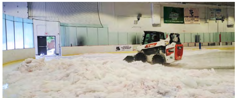
Bobcat removing ice from rink in slabs.
