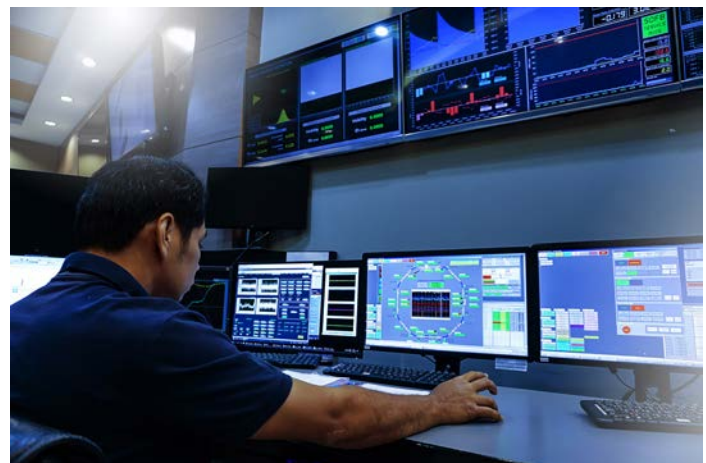
The Valmet D3 interface displays real-time process information in a complete, customer-oriented graphical HMI.
