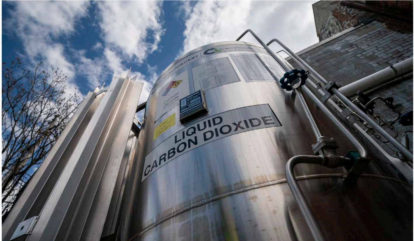
A liquid carbon dioxide containment unit stands outside the fabrication building of Glenwood Mason Supply Company, Tuesday, April 18, 2023, in the Brooklyn borough of New York. New York is forcing buildings to clean up, and several are experimenting with capturing carbon dioxide, cooling it into a liquid and mixing it into concrete where it turns into a mineral. (AP Photo/John Minchillo)
