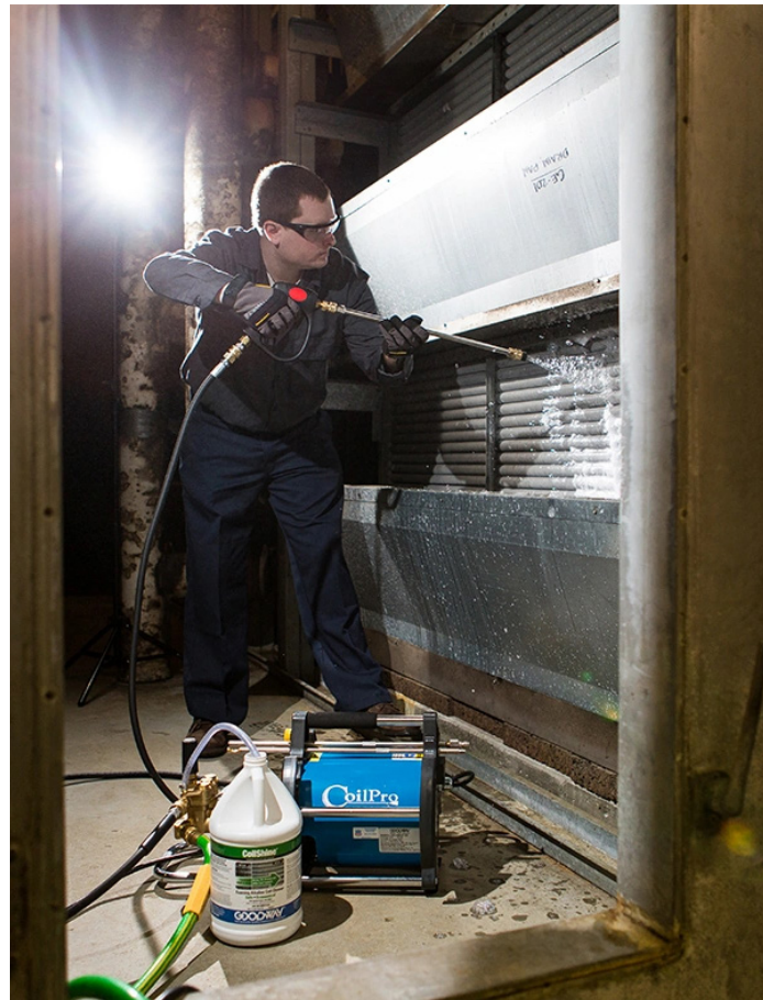
Use pressurized water to eliminate embedded dirt and debris.
