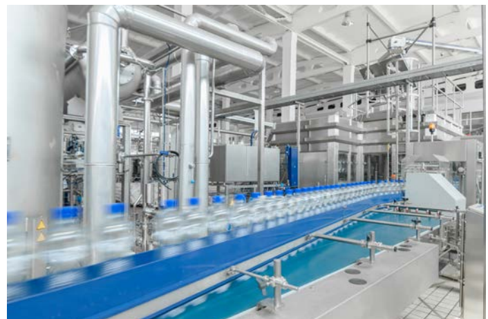
A DCS system serves as the hub of a processor’s operations and controls and monitors key variables such as flow, applied temperatures, pressure, level, and material conveying/handling.
