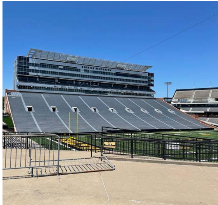
Western Specialty Contractors – Des Moines, IA Branch recently completed restoration and waterproofing of Nile Kinnick Stadium in Iowa City, Iowa.
