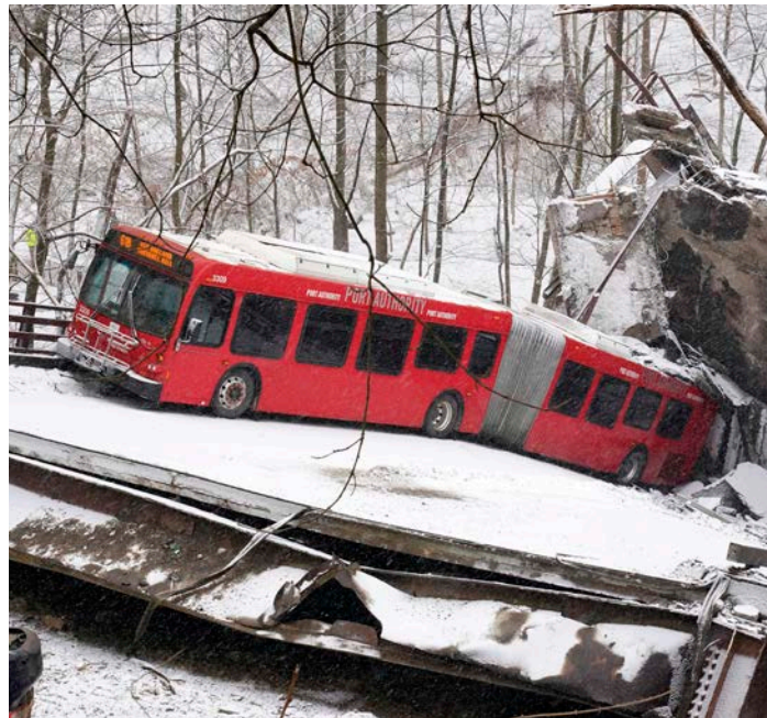
This is a Pittsburgh Transit Authority bus that was on the Fern Hollow Bridge in Pittsburgh when it collapsed in this file photo from Jan. 28, 2022. Investigators looking into the collapse of the Pittsburgh bridge last year want transportation officials nationwide to closely examine more than 10,000 other bridges with similar construction to make sure they don't have the same kind of corrosion that was found on the bridge that collapsed. (AP Photo/Gene J. Puskar, File)
