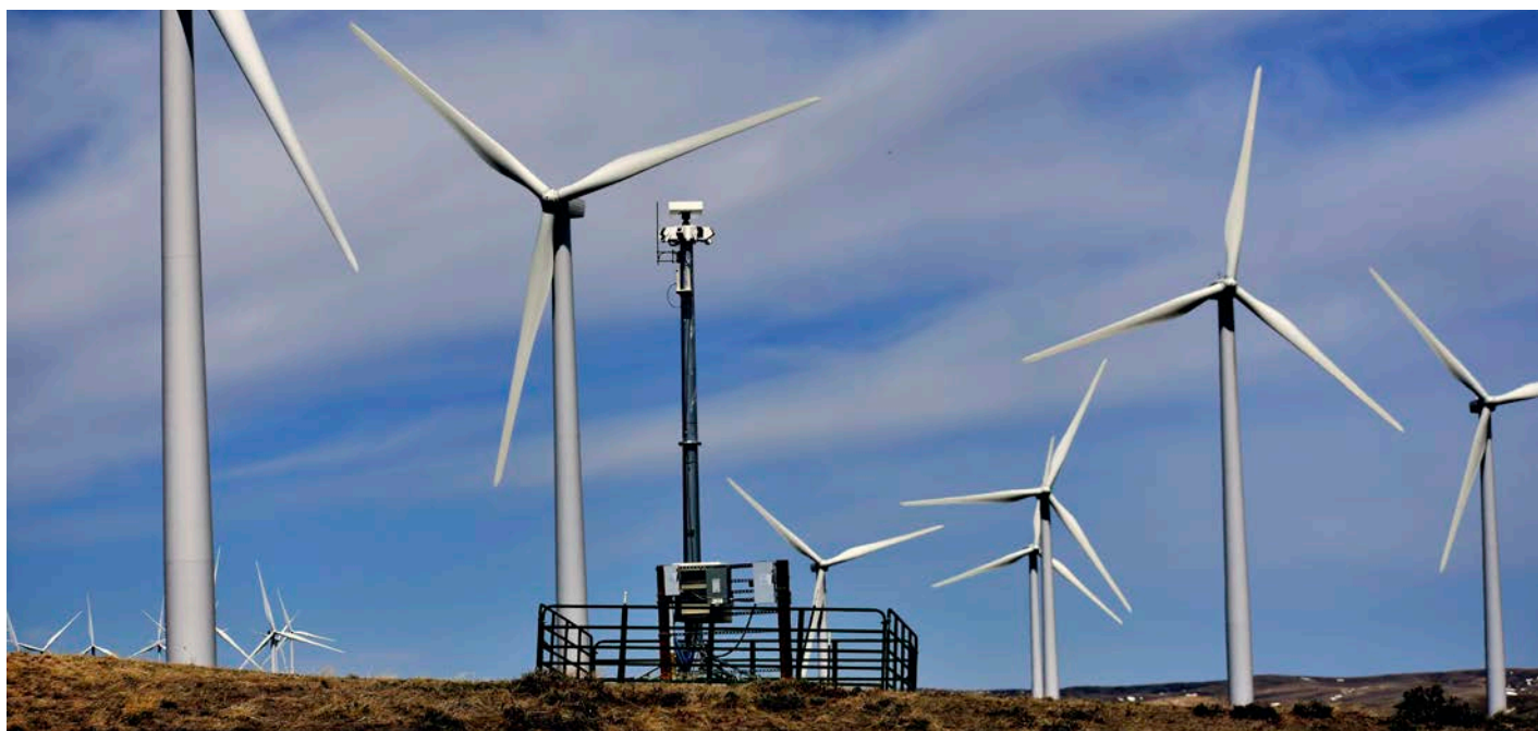
A camera system to detect approaching eagles is seen atop a pole at Duke Energy's Top of the World wind farm, on April 24, 2023, in Rolling Hills, Wyo. The company can shut down its huge turbines when eagles approach too closely, reducing but not eliminating fatal collisions after Duke was criminally prosecuted last decade for not adequately preventing eagle deaths. (AP Photo/Matthew Brown)
