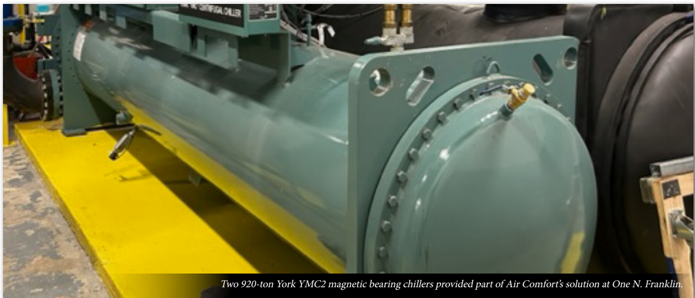
According to Air Comfort President Mike Devito, on average, a York YMC2 magnetic bearing chiller's payback period is reached within 5-7 years.
