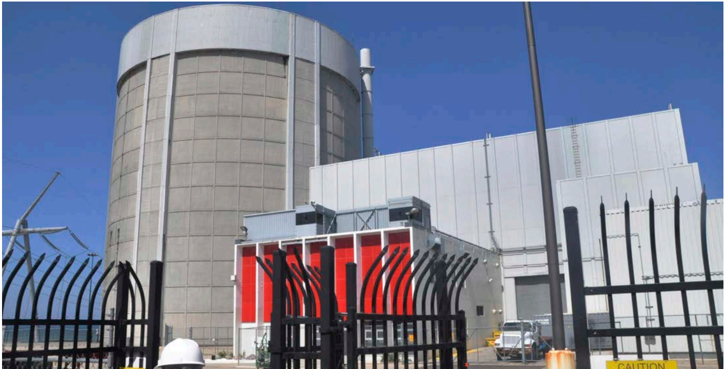
This June 24, 2010, file photo shows the Palisades Nuclear Generating Station in Covert, Mich. Holtec Decommissioning International, a company that tears down closed nuclear power plants wants to do in Michigan what has never been done in the U.S.: restore a dead one to life. Activists who long criticized Palisades as poorly maintained and dangerous don't want it resurrected. (John Madill/The Herald-Palladium via AP, File)
