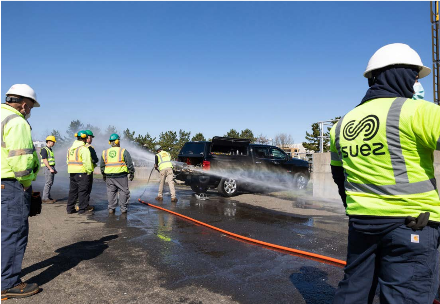
Sewer cleaning nozzles at extremely high pressures should only be used in a pipe - or the nozzle could whip around like a fire hose.
