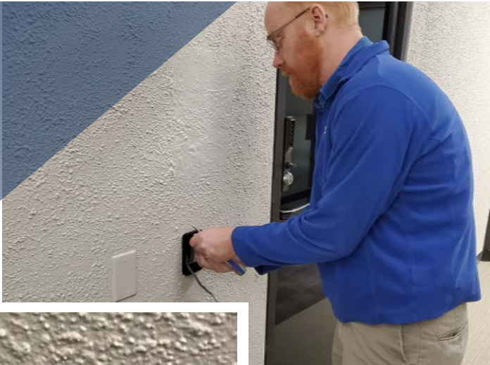
Installing a Bluetooth/smartphone-capable reader.
